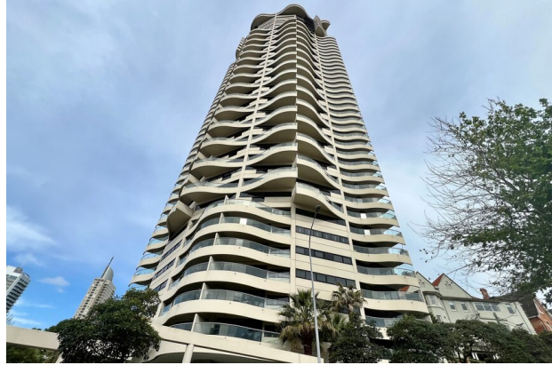
The 250-apartment complex the Horizon in Sydney has two public chargers for EVs. (ABC News: John Gunn)
